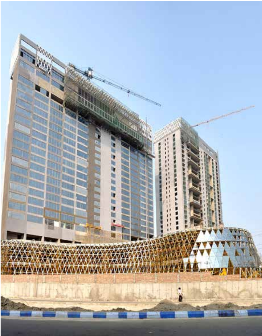
► JW Marriott Kolkata, under construction
