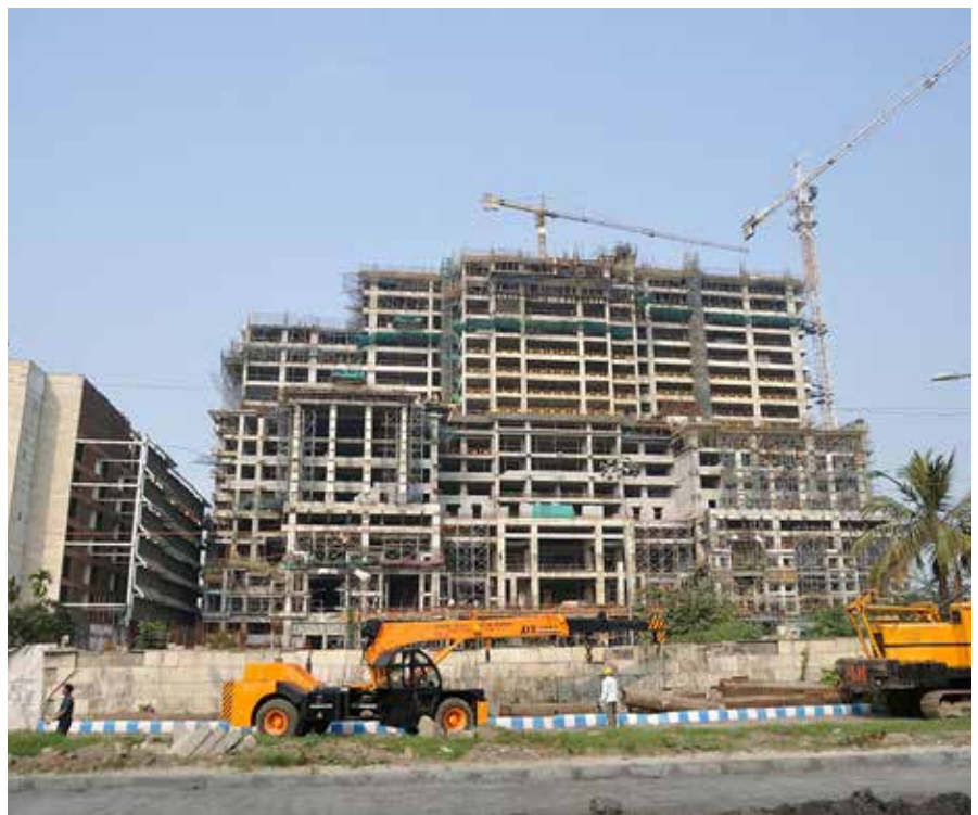
► Several projects are at different stages of construction in the city
