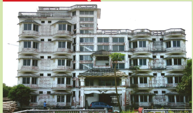
Niva Hotel Building
